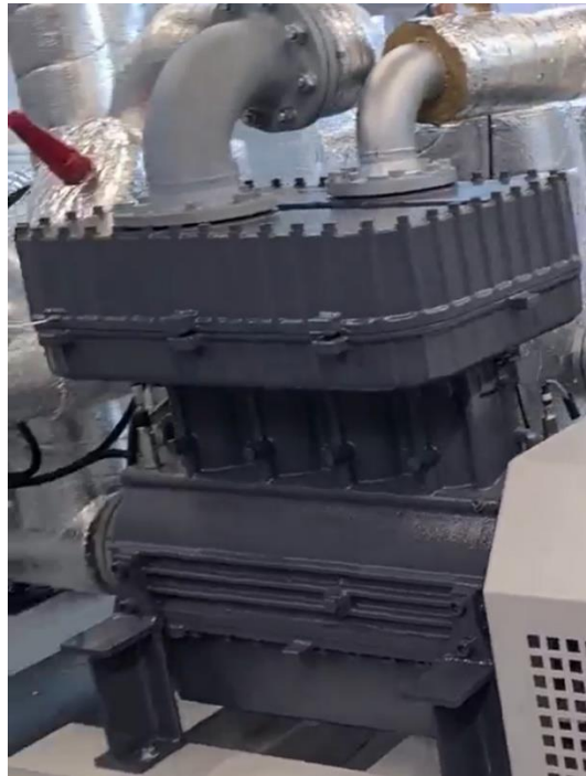
Figure 2 — The four cylinder piston compressor.
